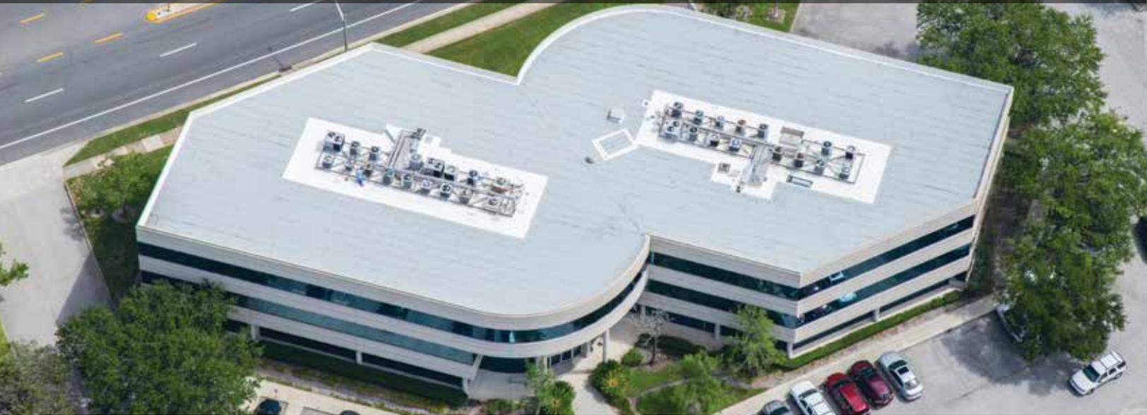
Parapro Roof Membrane provides an excellent solution for the area surrounding the air handlers on this Paradiene 20 TG/ 30 FR TG roof.
