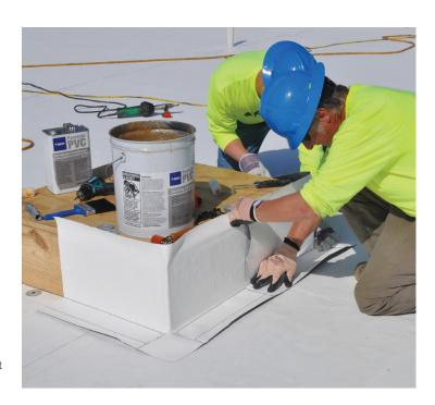
Prefabricated Parasolo PVC, KEE and TPX accessories are an efficient way to address detail conditions.
