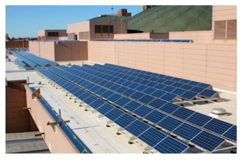
This photo is showing a large solar array that is mechanically attached to the structure at the corners and the quarter points along the leading edge.
