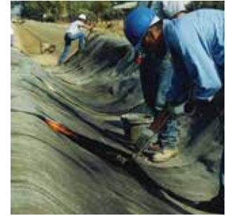
The simple torch welding technique used in Teranap installation helps to eliminate seam leakage problems.
