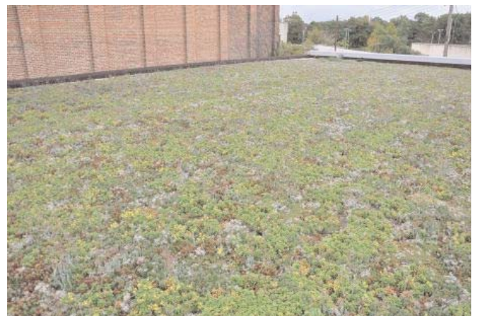
Photo 8 - One Year After Installation
