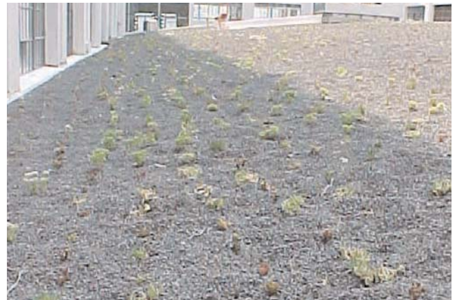
Photo 11 - Grown-on System after installation
