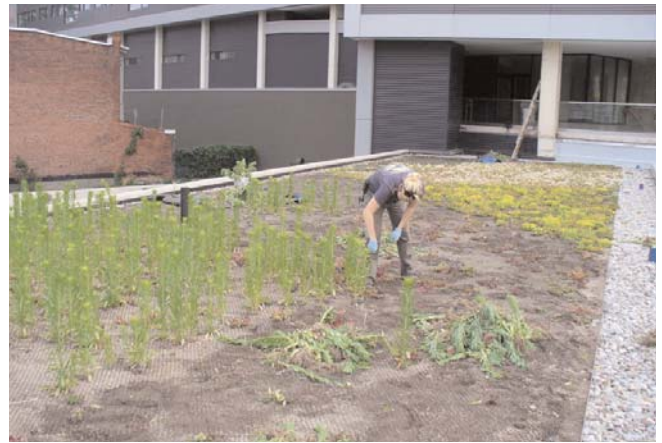
Photo 14 - Grown-on System 6 months following installation
