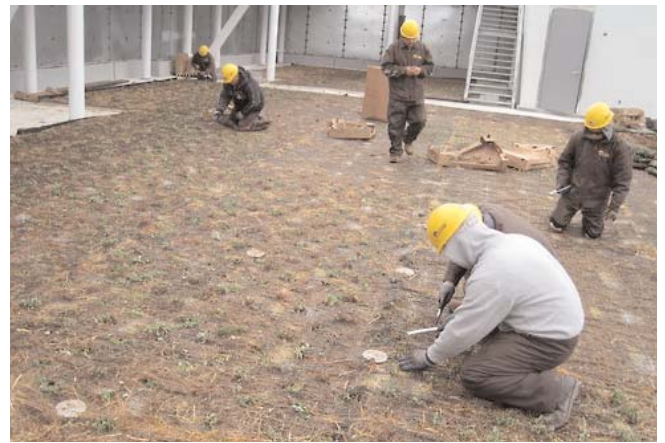
Photo 10 - Grown-on System during installation
