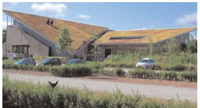
Photo 3 - Sloped Roof Application
